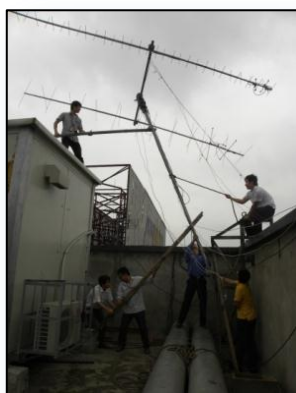
FIGURE 34: FSPACE TEAM BUILDING GROUND STATION FOR COMMUNICATION WITH LOW EARTH ORBITING SATELLITE, VIET NAM
